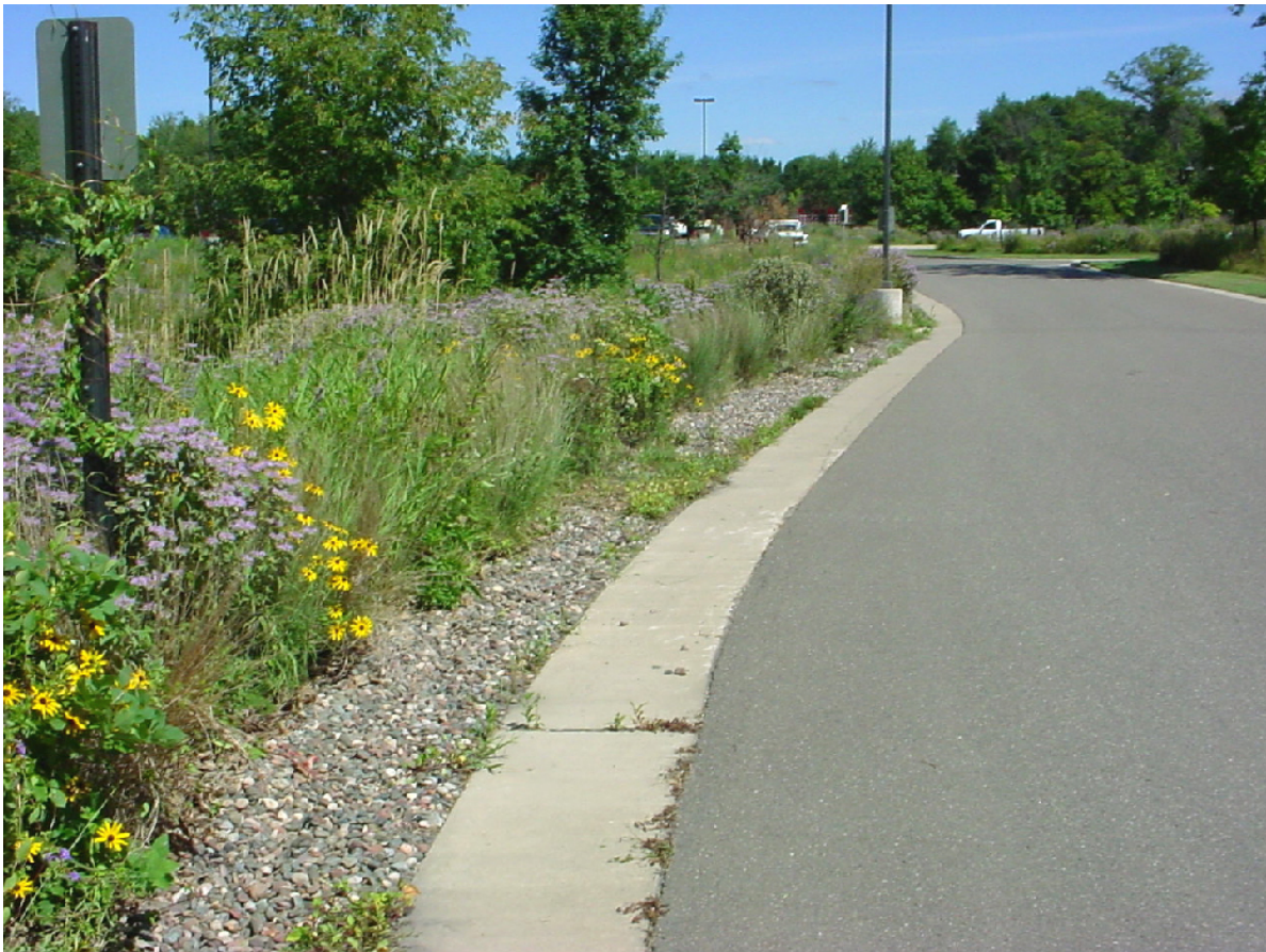
Figure 13. Photo of an infiltration trench in Lino Lakes, MN. Source: (17)
