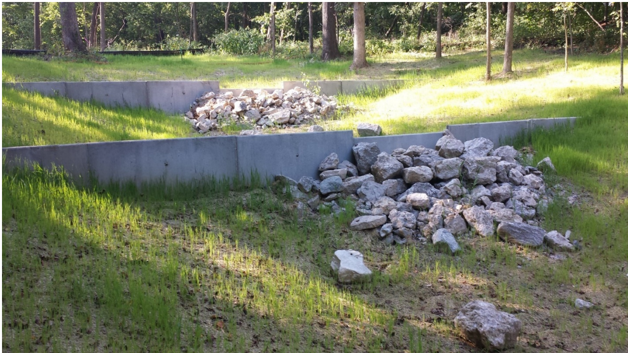
Figure 17. A grass swale with concrete check dams. Credit: LimnoTech. Source: (20)
