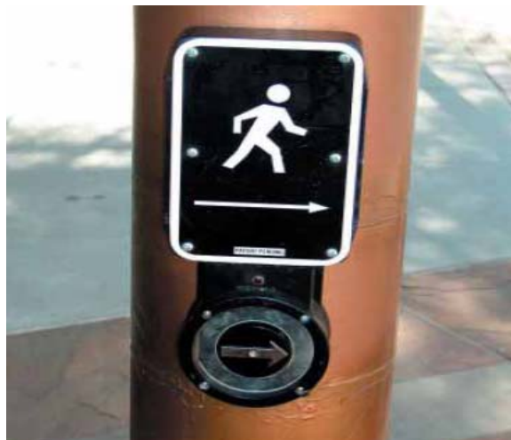
Figure 39: Accessible Pedestrian Signals
