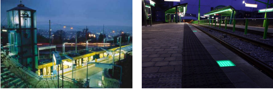
Figure 51: Light Rail and Complementary Pedestrian Walk Way with Lighting
