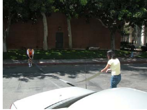
Figure 12: ILD being installed on the roadway
