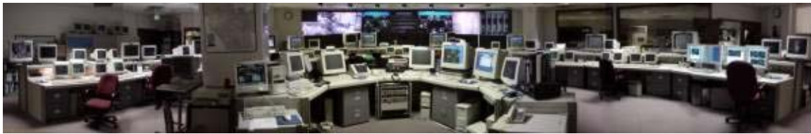
Figure 5: LADOT Traffic Surveillance and Control Center
