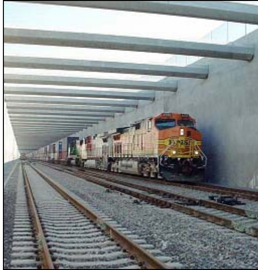
Photo shows a conventional double-stacked container train in the Alameda trench.
