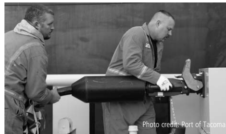
The first cargo ship at the Port of Tacoma is officially plugged in to a shore-side connection system in 2010 so that the vessel can shut down its diesel engines.
