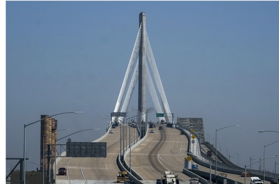
With three lanes in each direction, the bridge will be able to accommodate more truck traffic. The old bridge carried up to 16,000 trucks per day. Photo by Ringo Chiu.
