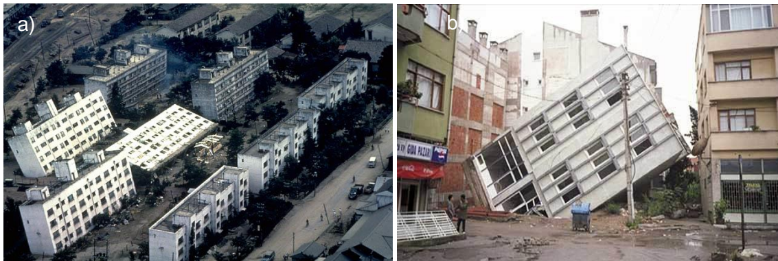
Fig. 2. a) Overturning failures in residential complex in 1964 Niigata earthquake, and b) Liquefaction-induced settlement due to loss of bearing capacity in 1999 Kocaeli earthquake (after NISEE 2016).
