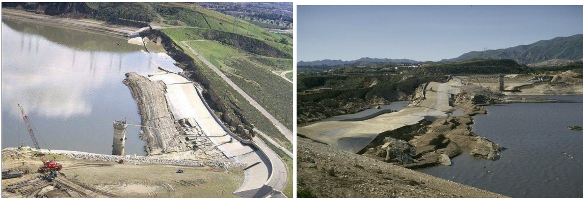
Fig. 5. Lower San Fernando Dam collapse due to San Fernando earthquake in 1971 (after NISEE 2016).
