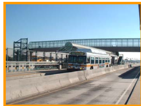
Figure 3.10: Platform level view
