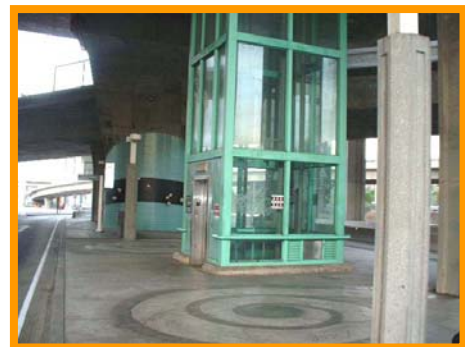
Figure 3.18: Platform Level View
