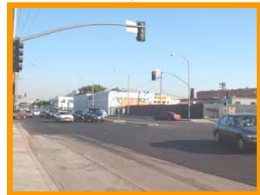
Figure 3.17: Neighborhood on the eastern side
