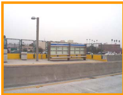
Figure 3.5: Platform level view of the station
